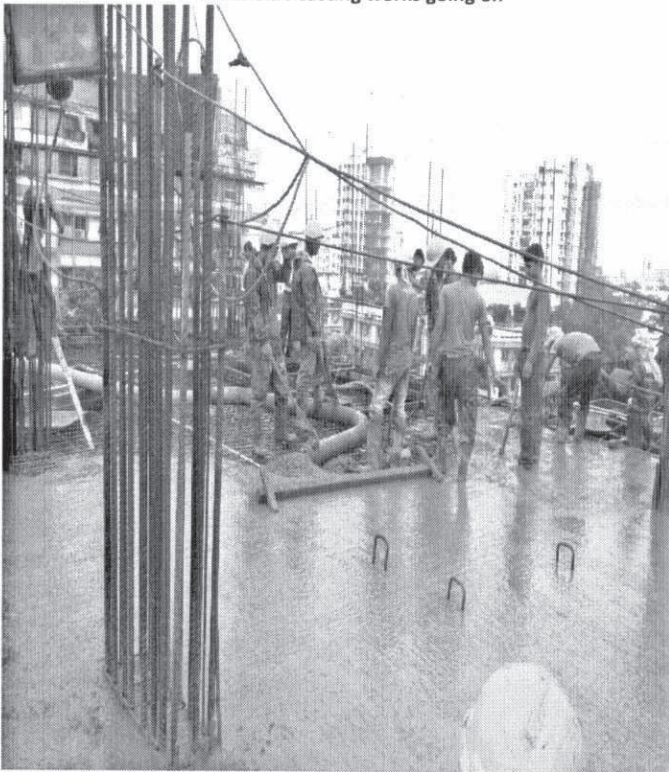
7 th Floor Slab casting works going on
