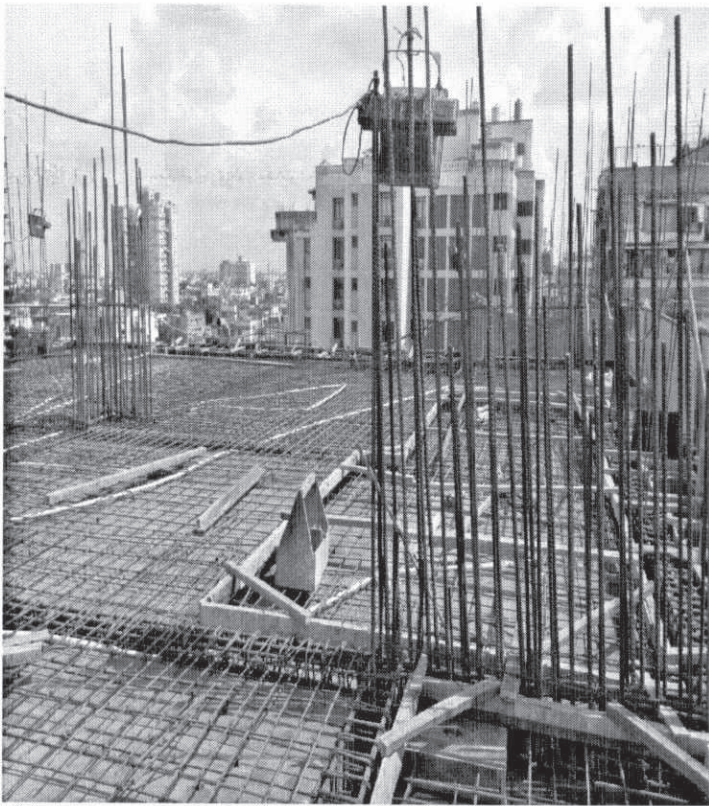
8 th Floor Slab part 1 Reinforcement works going on
