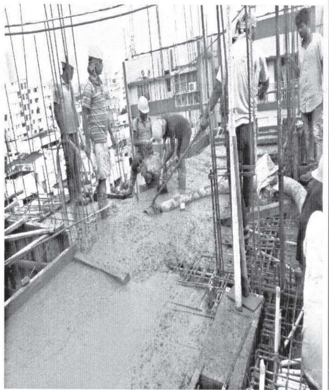
8 th Floor Slab Part-2 casting works going on
