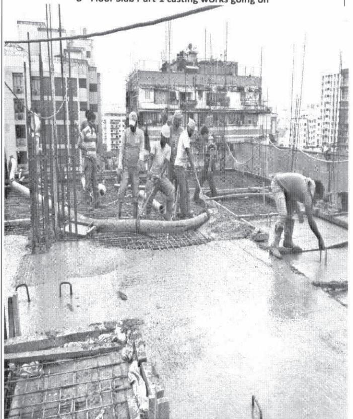
8 th Floor Slab Part-1 casting works going on
