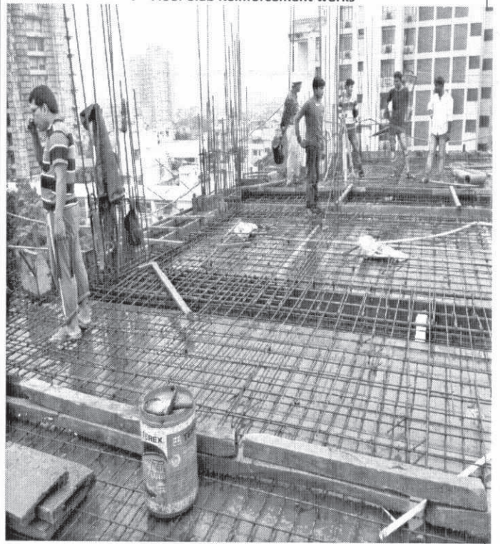
7 th Floor Slab Reinforcement works
